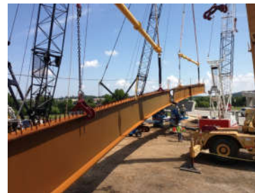
Fulbright Expressway, Fayetteville, AR
