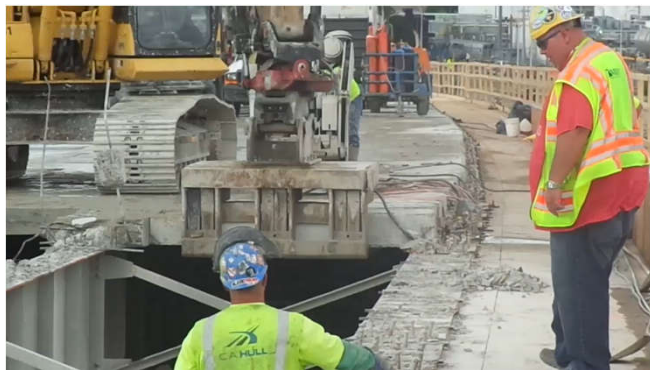
I-75 Deck Replacement, Detroit, MI
