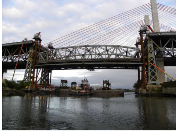
K Bridge Lift Span Demolition, New York, NY
