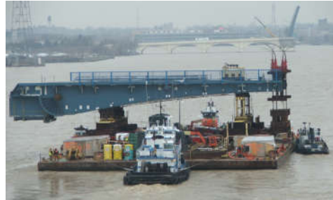
MLK Bridge Replacement, Toledo, OH
