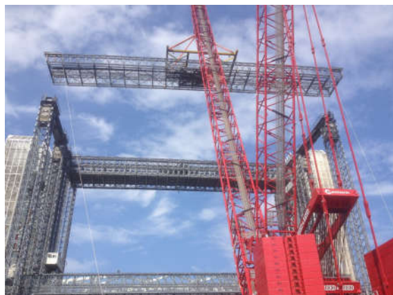
Fore River Lift Span Demolition, Quincy, MA
