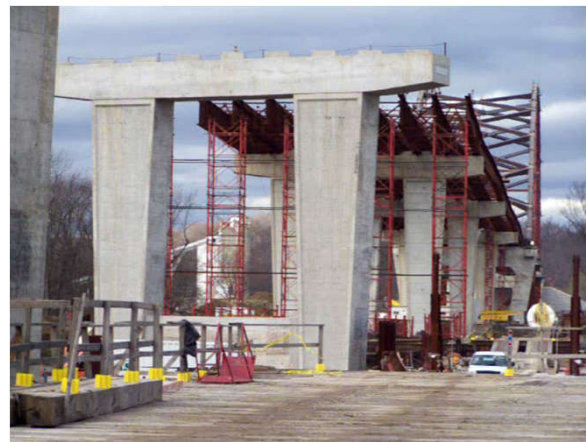
Blennerhasset Island Bridge, Parkersburg, WV
