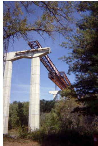
US 20 – Iowa River Bridge
