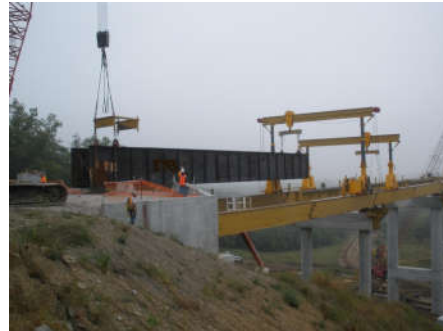
Kate Shelly Replacement Bridge, Boone, IA
