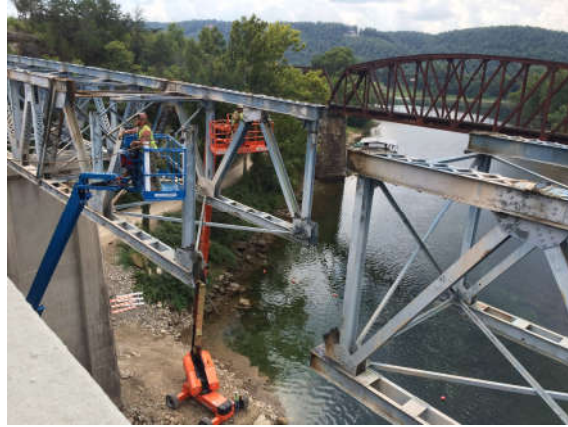
White River Truss Demolition, Prairie County, AR
