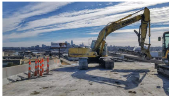
Lewis and Clark Viaduct, Kansas City, MO
