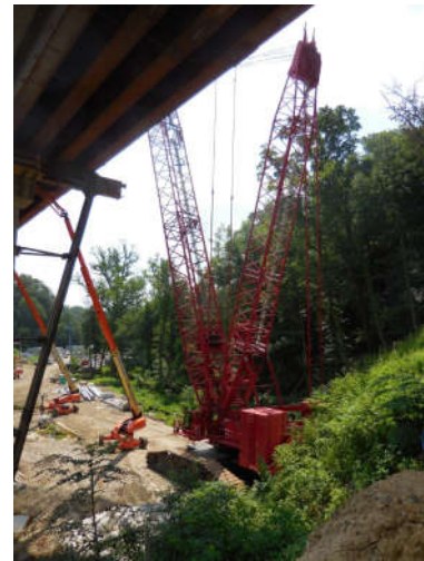
Crum Creek Viaduct, Swarthmore, PA
