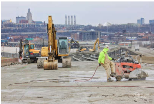
Lewis and Clark Viaduct, Kansas City, MO
