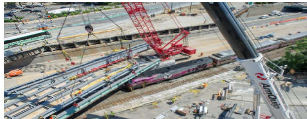
Comm Ave Bridge, Boston, MA
