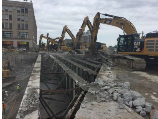
Comm. Ave Bridge, Boston, MA
