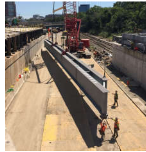
Comm. Ave Bridge, Boston, MA
