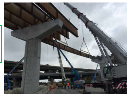
Gateway Interchange Flyovers, Johnson County, KS
