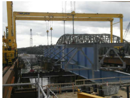
Whittier Memorial Bridge, Newburyport and Amesbury, MA
