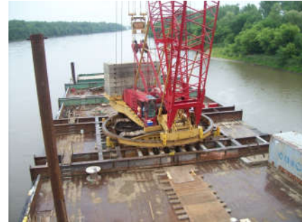
South Omaha Bridge – 4100 Ringer Crane
