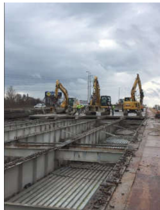
I-75 Deck Replacement, Detroit, MI
