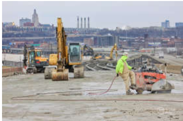
Lewis and Clark Viaduct, Kansas City, MO
