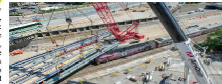
Comm. Ave Bridge, Boston, MA
