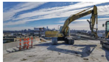
Lewis and Clark Viaduct, Kansas City, MO
