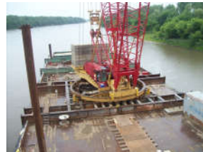
South Omaha Bridge – 4100 Ringer Crane
