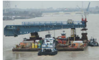
MLK Bridge Replacement, Toledo, OH
