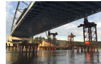
Whittier Memorial Bridge, Newburyport and Amesbury, MA
