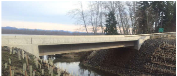
Mill Creek Bridge (Seradj, 2015)
