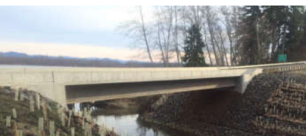
Mill Creek Bridge (Seradij, 2015)
