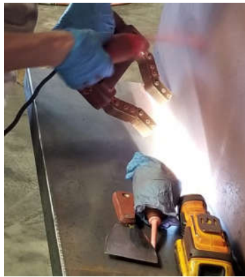
Magnetic particle testing (MT)
