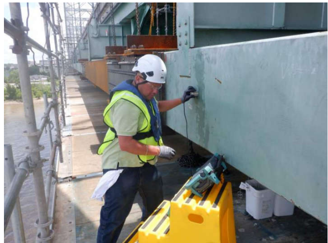
NDT Inspection of Arch Tie Member
