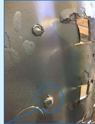
Shear stud weld failure
