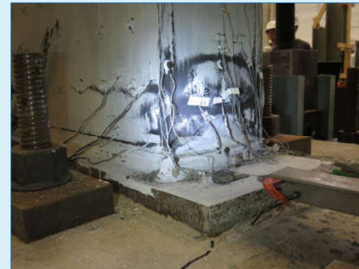
Local Buckling & Fracture During 4 \Delta y Cycles – Point D
