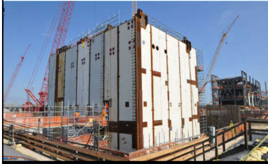
Vogtle Unit 3 CA20 Module June 2014 © Georgia Power Company
