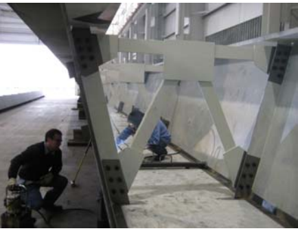
Cross Frames Used to Control Box Geometry
