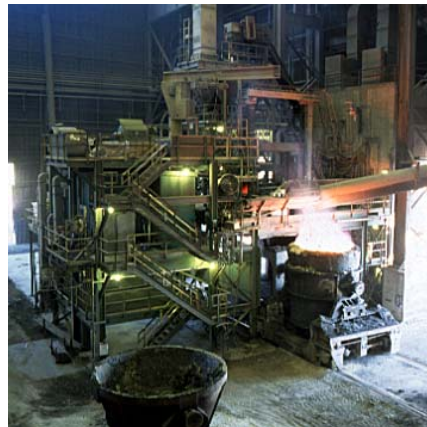
Ladle Metallurgy Furnace (LMF)
