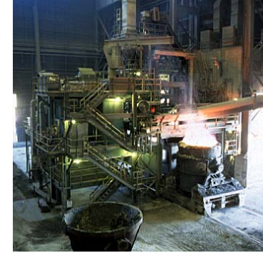
Ladle Metallurgy Furnace (LMF)
