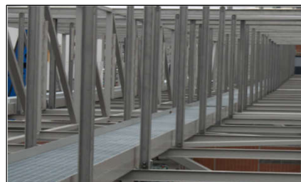
Pulp and paper plant © Outokumpu
