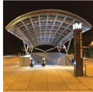
Stainless steel canopy over the entrance to Shady Grove underground station - one of 40 similar canopies on the Washington Metro
