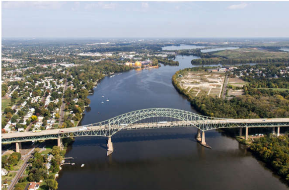
PA NJ Turnpike Delaware River Bridge
