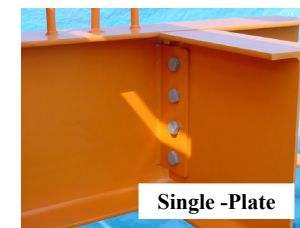
Single-Plate at HSS Column
