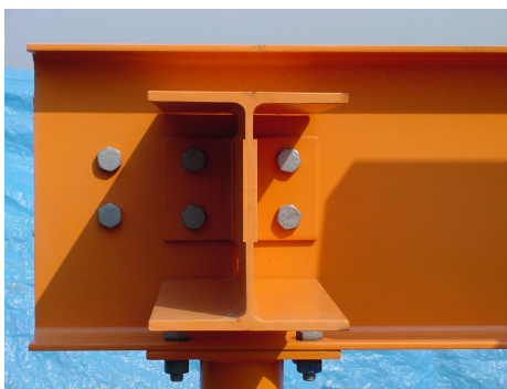
Beam Dropped for Joist Seat
