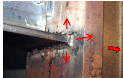
Example: Beam flange to (thick) column flange T joint
