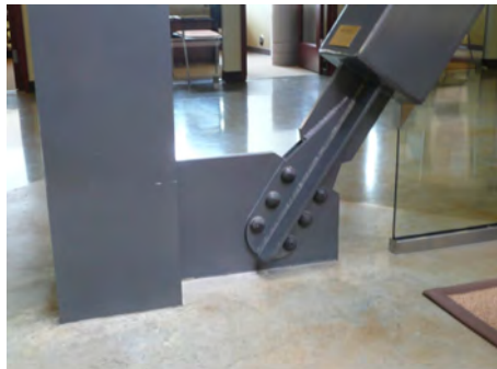
Direct bolting of core
