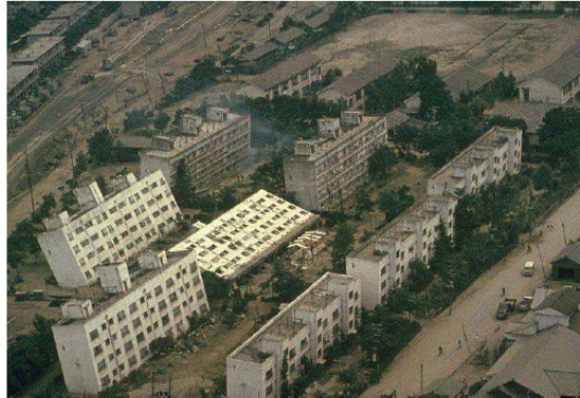
Fig. 1-8. Settlement in apartment buildings due to soil liquefaction, 1964 Nigata, Japan, earthquake. (Photo courtesy of University of Washington)
