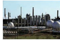
Risk Category IV: Hazardous facility
