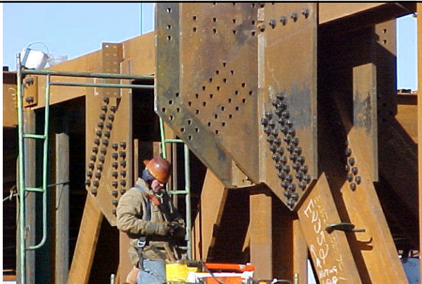
“Pinned” Truss Connections
