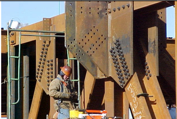
“Pinned” Truss Connections
