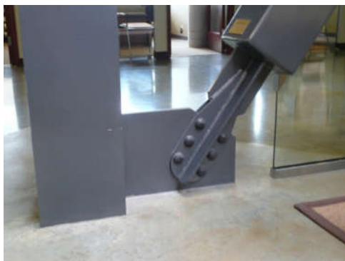
Direct bolting of core
