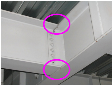
Lateral bracing provided by concrete structural slab and full-height perpendicular framing
